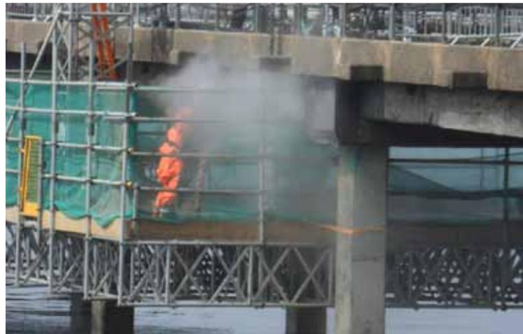
RGL proposed an innovative technical solution which employed a low flow ultra high pressure water jet. By increasing the pressure up to 2,500bar it enabled RGL to halve the water flow required. This resulted in a manageable and permissible reaction force on the operators. This low reaction force meant that operators suffered less work fatigue and it also reduced the risk of injury and accidents.
